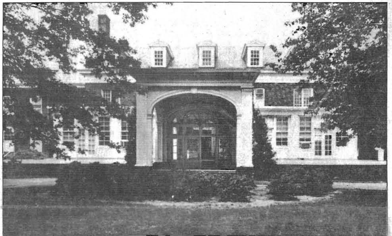
ORGINIAL COURSE: The orginial Bellerive Country Club— before it became part of the UM-St. Louis campus. Sitting behind the now demolished building currently is the Thomas Jefferson Library.
